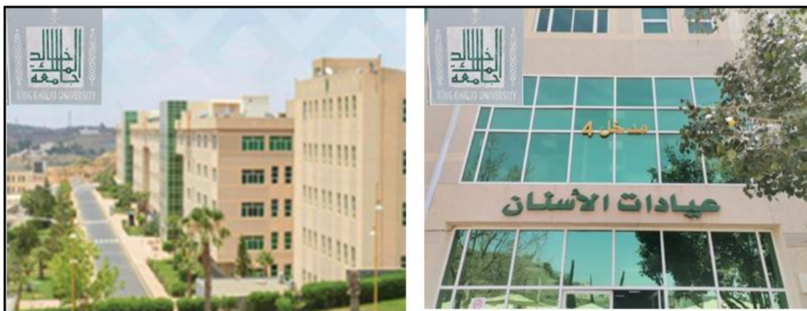
Figure 1.2 Main building of College of Dentistry, King Khalid University, Abha city, Asir province. ( https://www.kku.edu.sa/en/node/2821 ), accessed June 2022).
