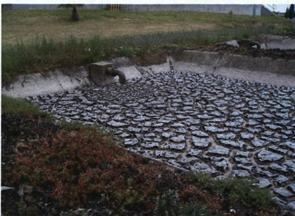
IX. Dry bed (Sewage sludge allows to be dried before removal)
