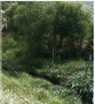
VIII. Outlet just outside WWTW (Final effluent discharges into the river)
