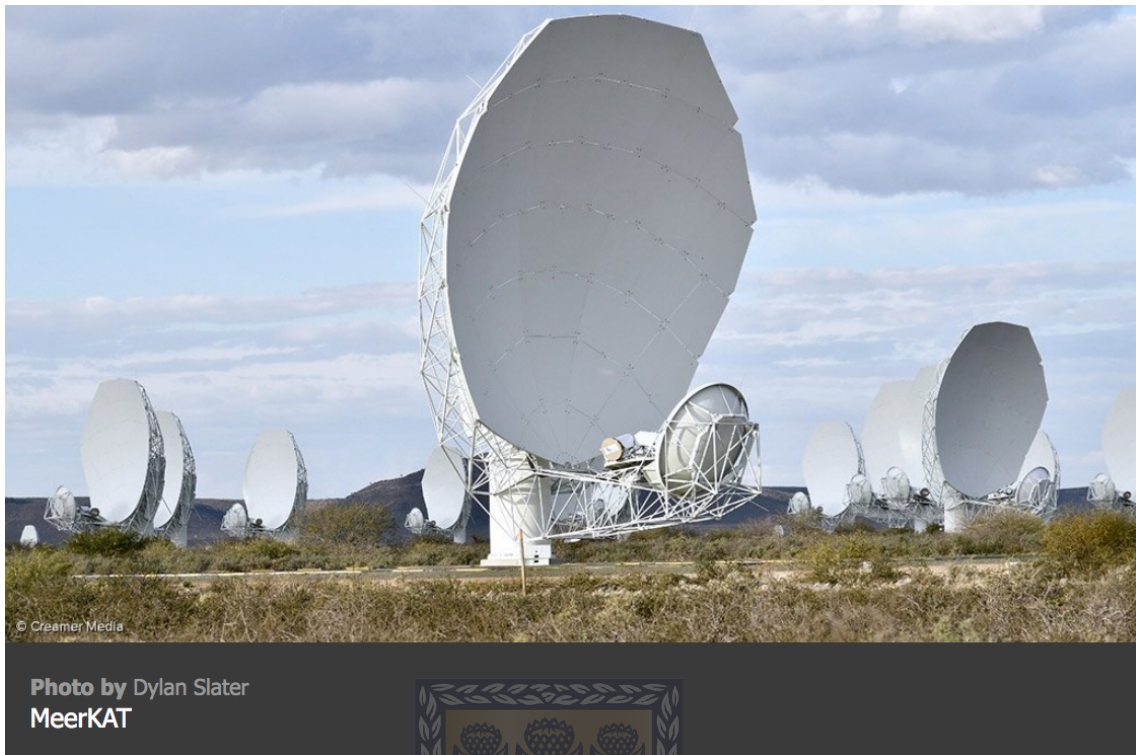
Figure 3.5: Image of the MeerKAT dishes located in the Karoo desert in South Africa. We can see the Gregorian design characterised by the offset of the secondary reflector. This configuration maximises the collecting area, as it does not block the aperture. At the heart of each dish is a receiver tuned to the L-band (900-1670 MHz) with 4096 channels, which are some of the most sensitive arrays ever created. Image taken from the MeerKAT webpage.
