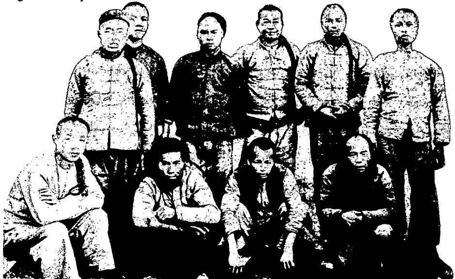
Some of the first Chinese workers to be brought to the Rand to ease the shortage of labour on the mines.
