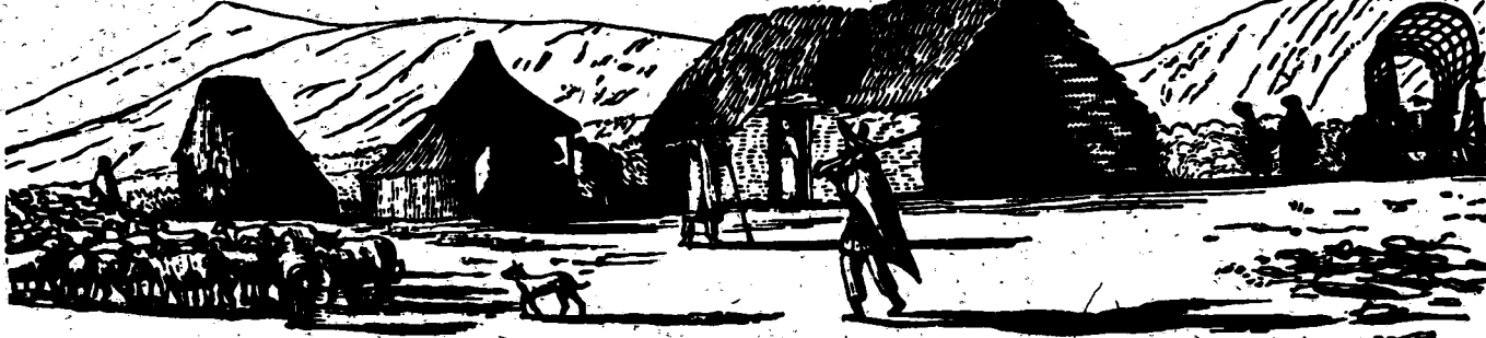
A settler farm in the early years of colonialism, using slave labour.
