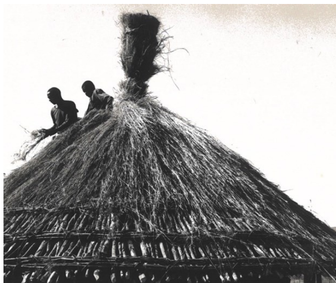
Figure 2.24: Making of a thatch roof. The sheaf, before spreading in van der Waal's "Die Woning en Woonwyse onder die Venda" (1977)
