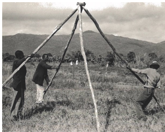
Figure 2.22: The four longest roof posts are set up, in van der Waal's "Die Woning en Woonwyse onder die Venda"
