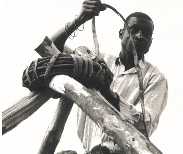
Figure 2.23: The ring around the five main posts of the roof is reinforced with bark, in van der Waal's "Die Woning en Woonwyse onder die Venda" (1977)
