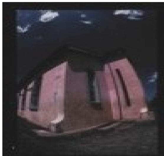
Figure 2.12: Photograph from sheet 3, 1970s.
