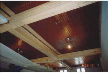
Figure 4.19: Stepping Stones classroom and entrance were reconfigured as the District Six Museum Memorial Hall. Columns were removed and I beams installed to support the ceiling to provide an open plan design. Photographs Rennie Scurr Architects.
