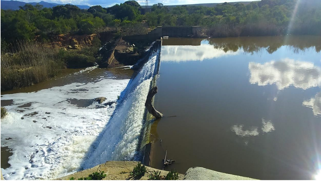
Figure 3.5 Weir at Nacht Wacht Farm which acts as a broad crested flow measuring weir
