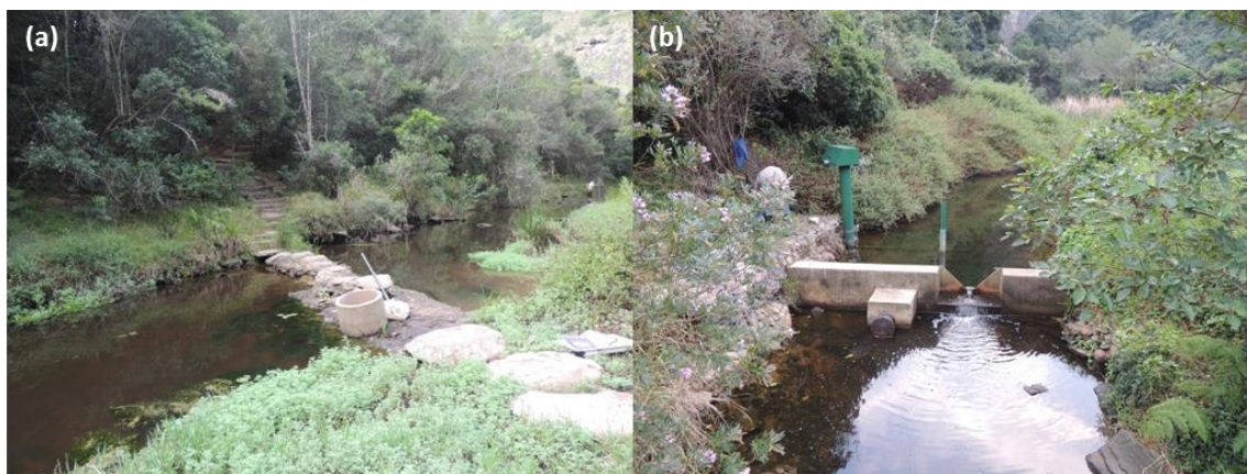
Figure 2.11 Instream obstructions at site K4 on the Duiwe River (a) shallow causeway for river crossing, looking downstream and (b) DWS gauging weir and water quality monitoring point, looking upstream
