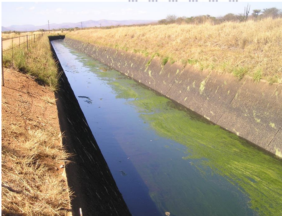
Figure 6.1 Show long strings of filamentous algae in extreme cases up to 10 meter in length in the Loskop irrigation canals.
