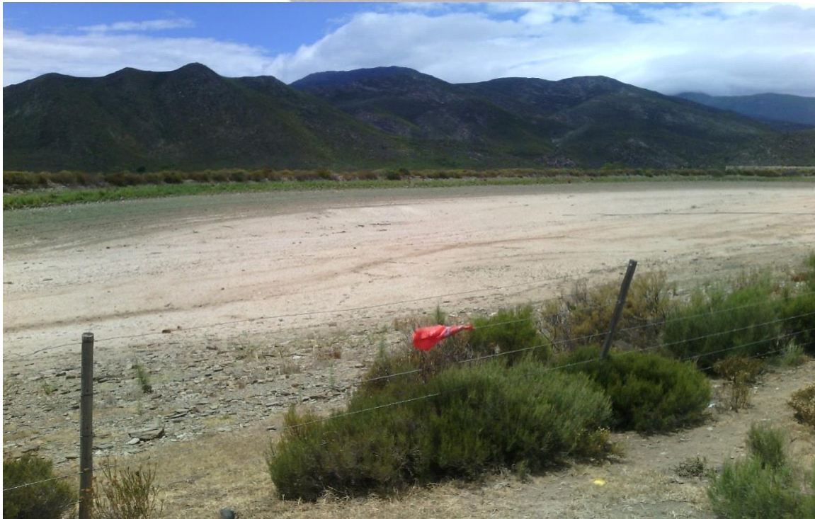
Figure 4.3: SSFs' Dam during dry season (taken on 31st January 2015)
