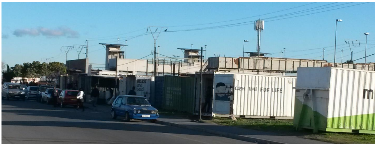
Figure 8: Small Business Centre at the Heideveld Station in Gugulethu
