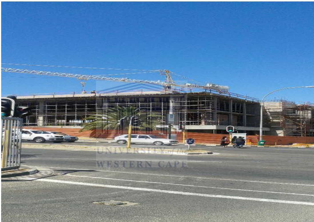
Figure 5: Panorama Hospital Project
