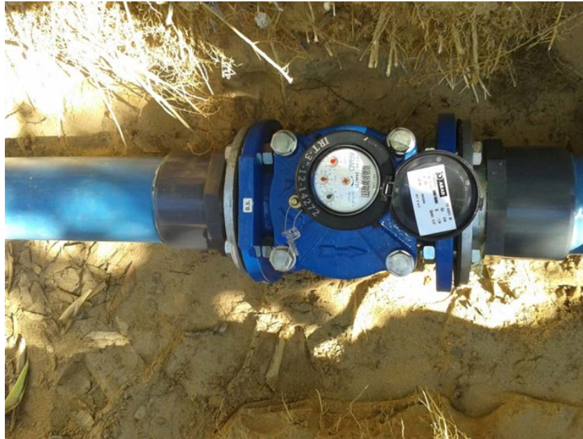
Figure 4.2: Flow meter installed at Patrysborg Farm to measure water that was used in the packhouse for 2013/2014 Navel orange.
