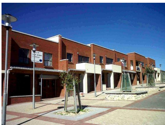
Multi Purpose Flats at Harare
