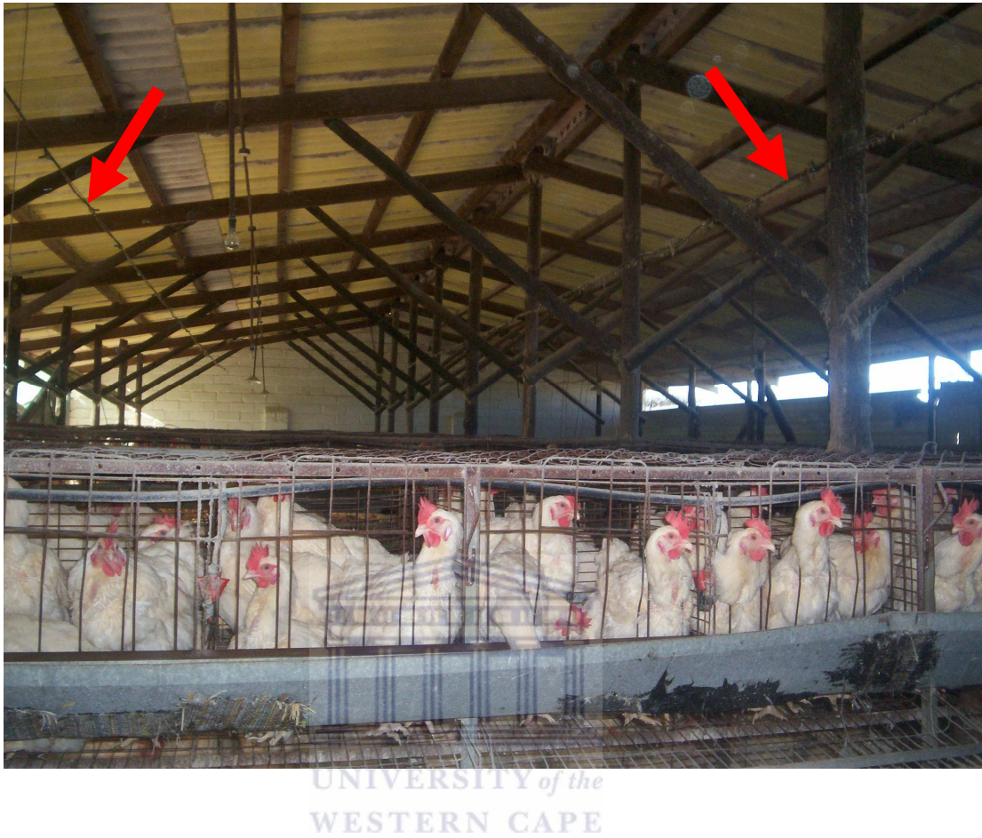
Figure 3.2: Photograph of the poultry set-up: The pipes for biocide dispersal can be seen above the pens.
