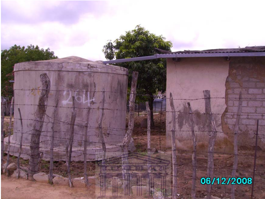
Insert/plate 5.6: World Vision funded rooftop harvesting tank in Enable. The number 264 stands for the 264th beneficiary from the World Vision funded project in the village.
