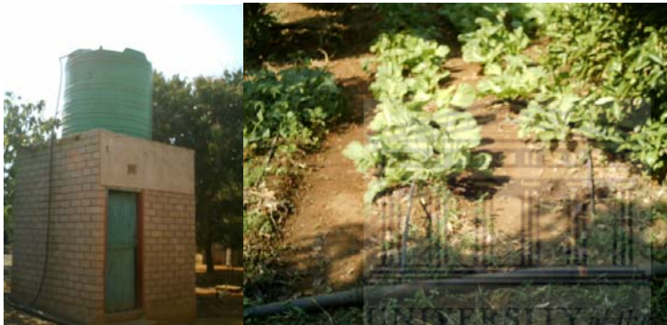
Insert/plate 5.2: Borehole pumphouse and storage tank, and drip irrigation in Lorraine
