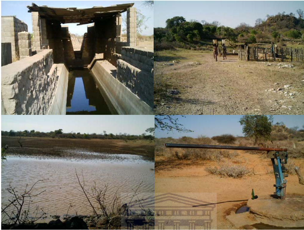
Insert/plate 4.2: Some communal water infrastructure in Manama, Ward 17
