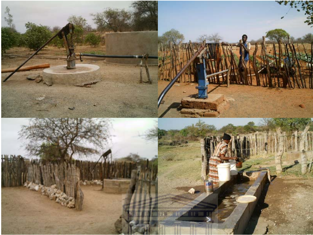
Insert/plate 4.3: Private boreholes for multiple uses - domestic, irrigating garden, brickmaking enterprise, and sharing with neighbours and close kin. The type of fencing shown is used for protection against vandalism by livestock and other villagers.
