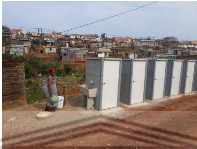
Figure 2.8 Mossel Bay NUSP ISSP 23 informal settlements UISP Project 2019 (Source: Zutari, 2023).
