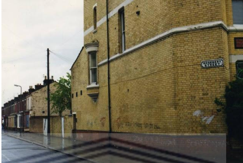
Figure 3: Rosebery Street from Princes Avenue before demolition, M.P. Ashworth, “The QuarryMen, Rosebery Street and King John,” (Accessed 17 October 2023)
