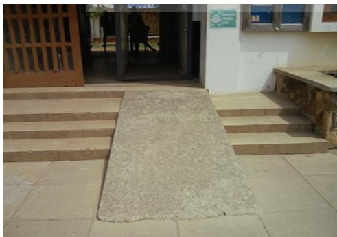
Figure 5. 38: A ramp with no handrails on both sides at one of the university libraries, UL1 (Source: Field data, 2022)
