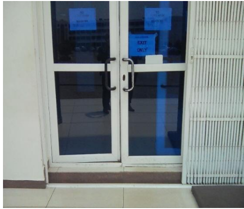
Figure 5. 42: An entrance gate with a threshold in one of the university libraries (UL9) (Source: Field data, 2022)
