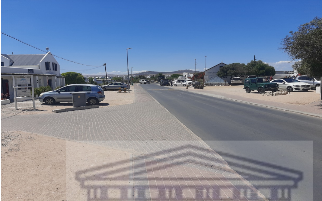
Figure 3: Upgraded roads in Paternoster
